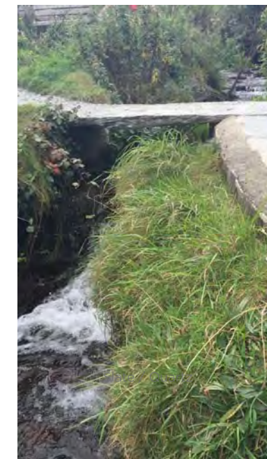
Slate beam bridge
