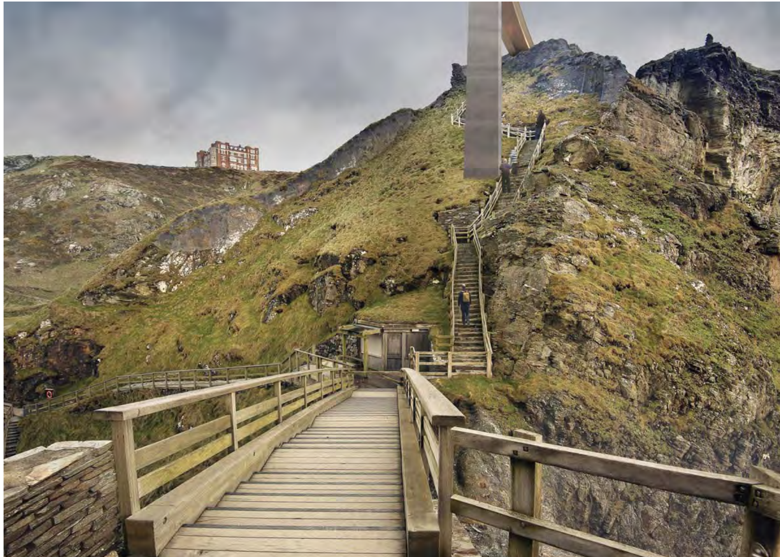
At the bottom of the ravine
