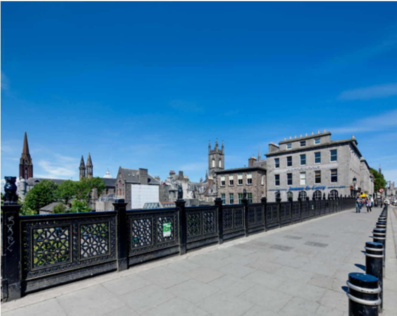
FIG 10: View from Union Street looking northeast.
