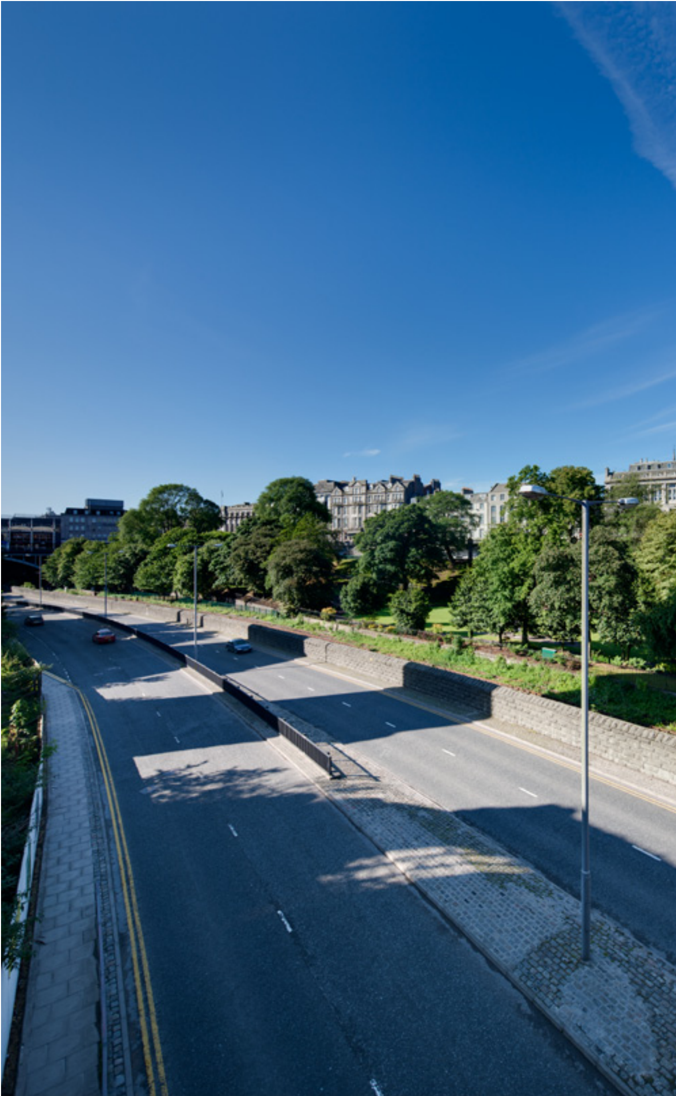
FIG 14: View from eastern end of Rosemount Viaduct looking south
